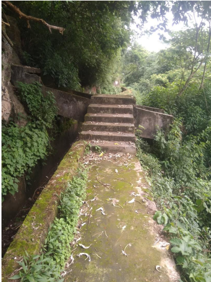
Figure 2 Showing Overhead Drain from Houses in Mawprem and Power Channels of the Sonapani Mini Hydel Project
