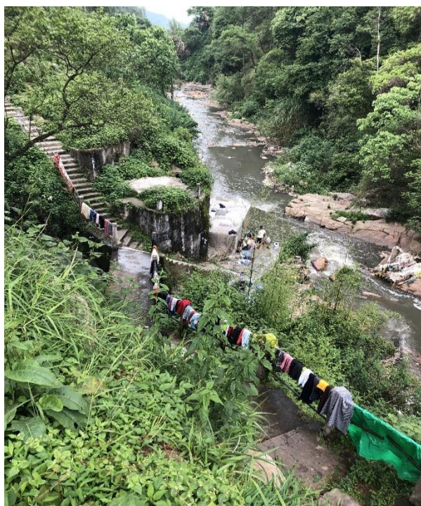
Figure 1 Public Washing Area at the Sonapani Mini Hydel Project Site
