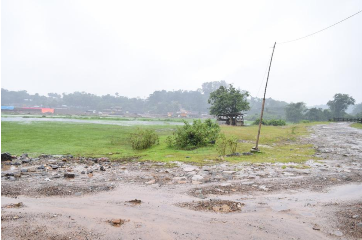
Figure 4 Dawki - Muktapur Road which passes through project site
