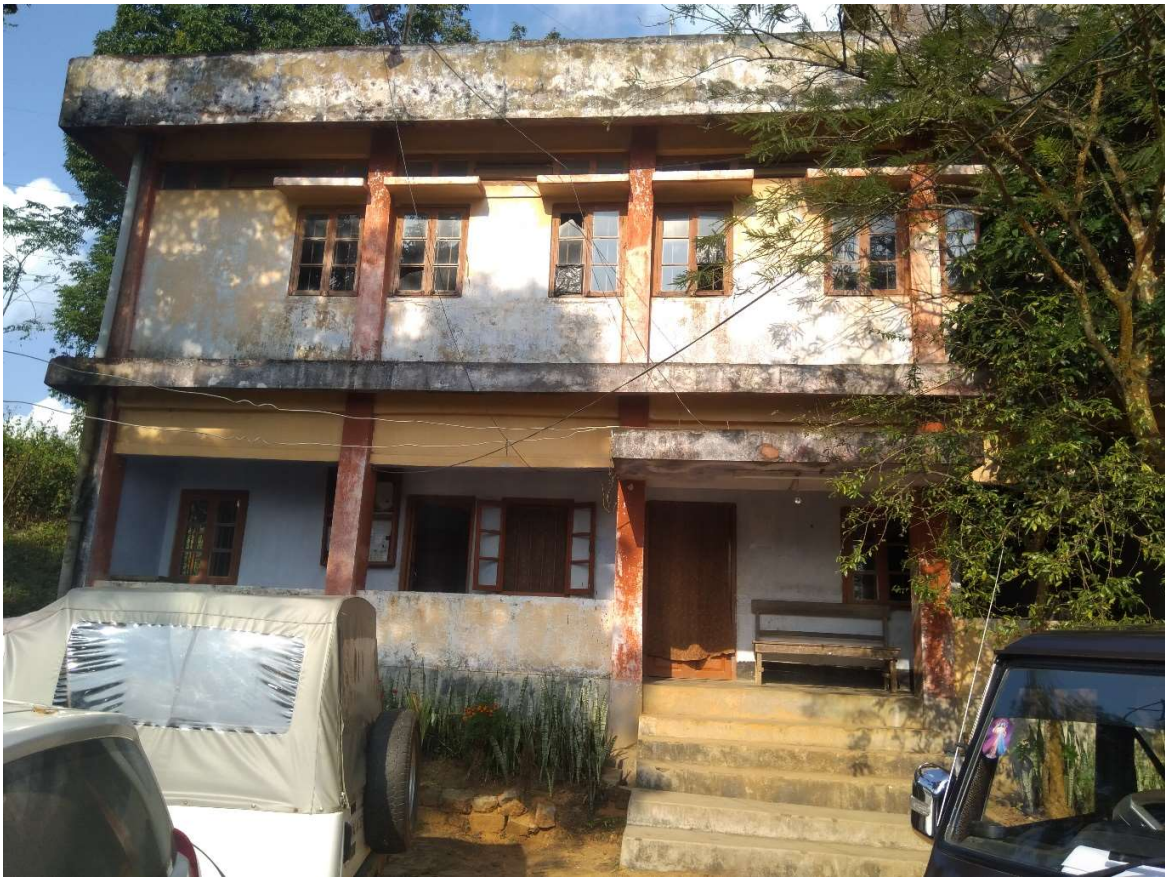
Figure 1 Existing Sub-Fire Service Station Office
