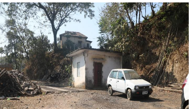
Old weigh bridge to be dismantled
