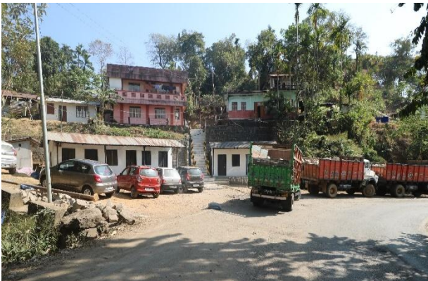
Individual houses to be affected
