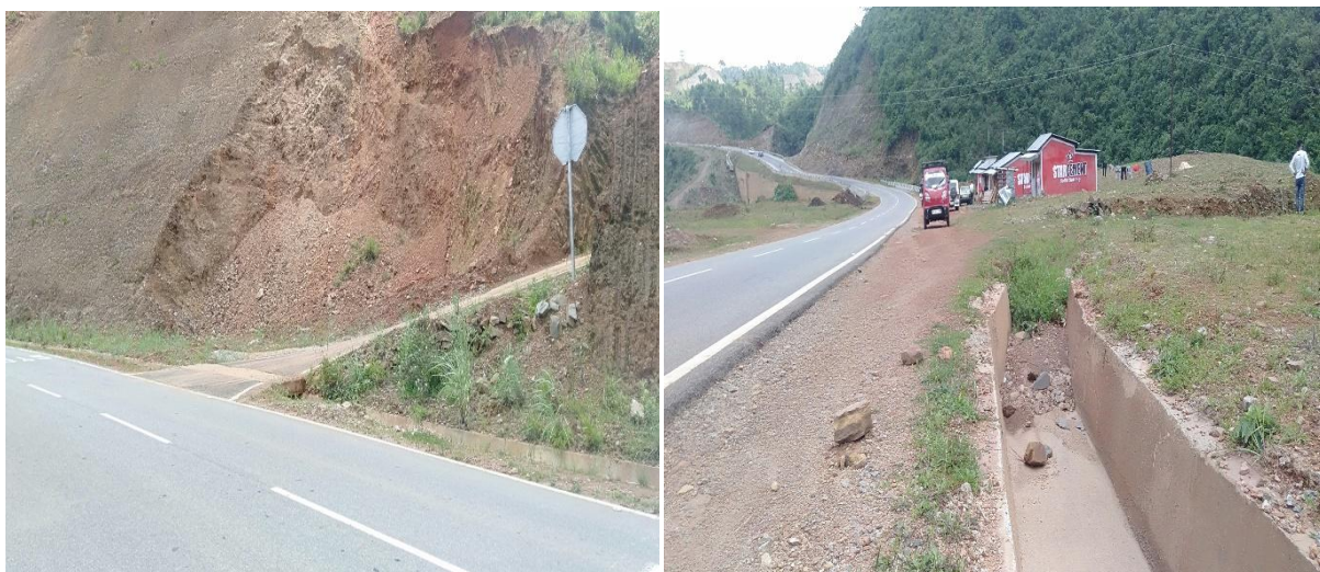
Figure 3: Site visit in Lwai village
