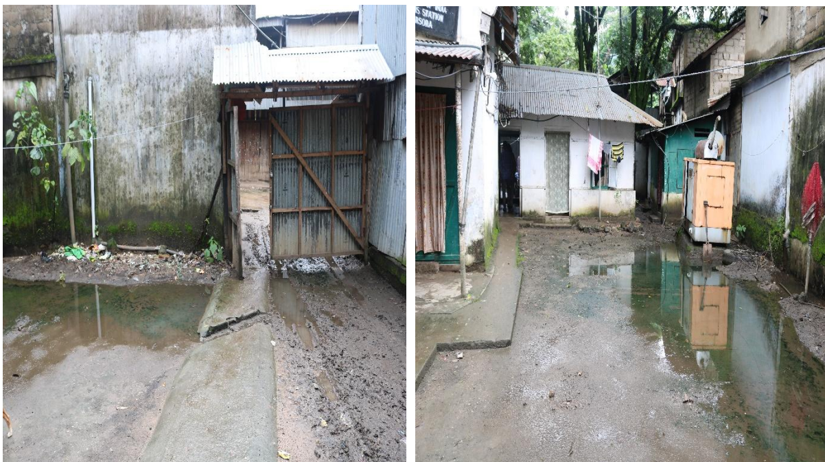
Figure 3: Pictures indicating the need for land acquisition for Borsora Customs Office
